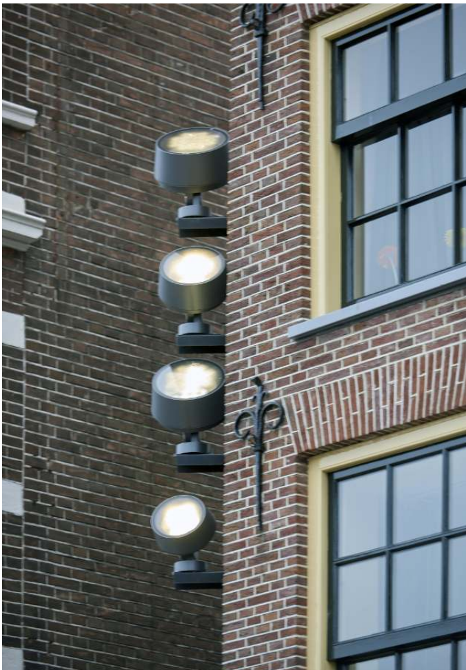
Wijnhuistoren, Zutphen. Lighting design: Studio DL, Hildesheim. Photography: Thomas Mayer, Neuss.
