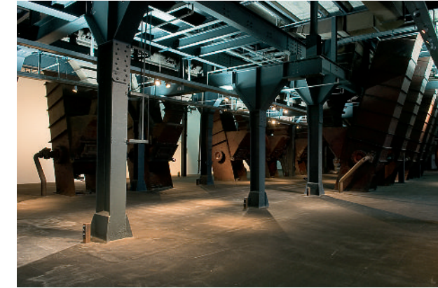
The lighting concept for the exhibition areas in the coal washing plant at the Zollverein colliery in Essen uses fluorescent light in daylight hues as indirect lighting for the ceiling. This is combined with warm-toned accents from spotlights with low-voltage halogen lamps.
