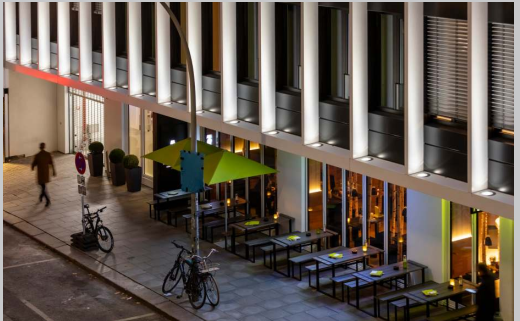
Facade of Brand-sende office building, Hamburg. Architecture: Akyol Kamps, Hamburg. Lighting design: Akyol Kamps, Hamburg. Photography: Frieder Blickle, Hamburg.
