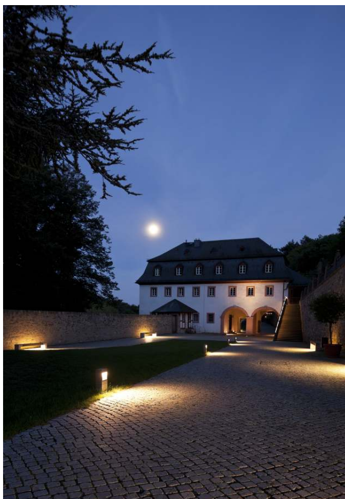
Eberbach monastery, Eltville. Architect: Rimpl + Flacht Architekten, Wiesbaden. Lighting design: Ing. Bamberger, Pfünz.
