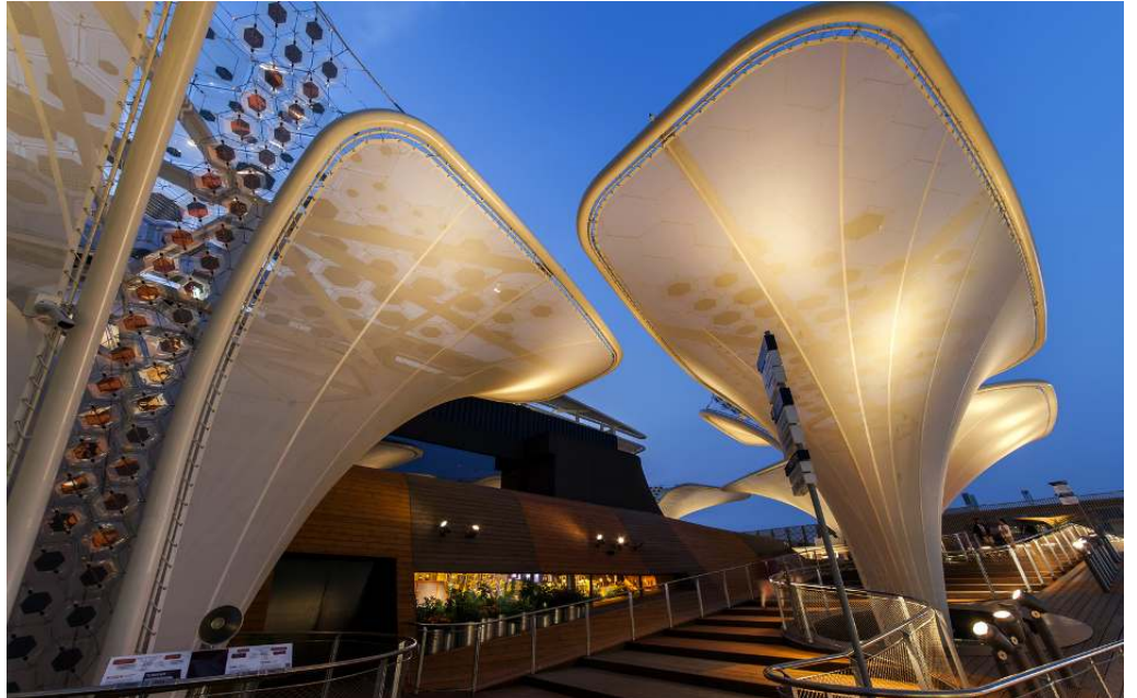
German Pavilion "Fields of Ideas" at the EXPO 2015, Milan. Concept: Arbeitsgemein- schaft Deutscher Pavillon GbR; Milla & Part- ner, Stuttgart; Schmidhuber, Munich; Nüssli GmbH, Roth. Exhibition design: Milla & Partner. Architecture: Schmidhuber; Nüssli. Photogra- phy: Dirk Vogel, Dortmund.
