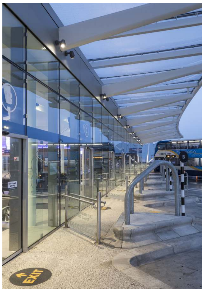
The Hard Interchange, Portsmouth. Architecture: AHR Architects, London. Lighting design: Lachman Consulting of Leeds. Photography: Lukas Palik, Düsseldorf.
