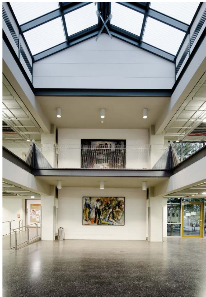
University of Neubrandenburg, Building 4, Neubrandenburg / Germany. Architecture: A&S GmbH Neubrandenburg. Lighting design: NEIB - Neubrandenburger Elektro-Ingenieur-Büro GmbH. Installation: EIM GmbH Elektro-Installation-Montage, Greifswald. Photography: Frieder Blickle, Hamburg.
