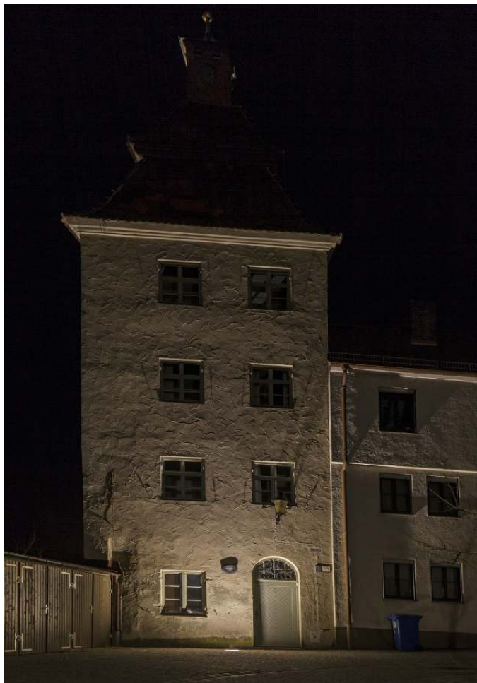
Ursula Tower, Günzburg. Lighting design and E-planing: Conplaning GmbH, Ulm. Photography: Dirk Vogel, Dortmund.
