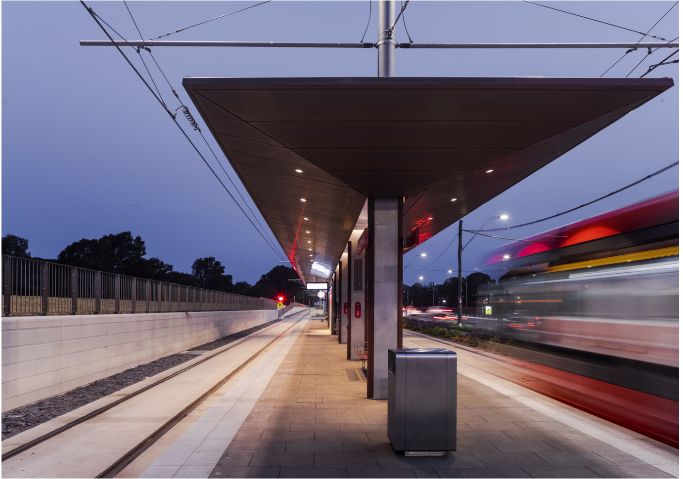
Sydney Light Rail, Sydney. Architecture : Grimshaw. Conception lumière : Electrolight, Sydney. Photographie : Jackie Chan, Sydney.
